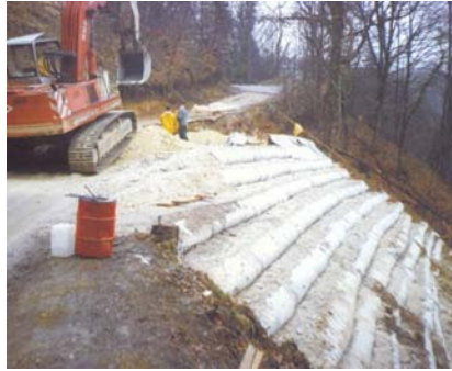
Figure 7. Construction of the reinforced soil structure (Polyfelt, 2002)
