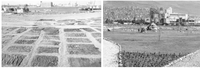
Figure 1. Application of geotextile and lay out of crushed stone in Melez Delta and the final view (İBB, 2001, Yılmaz et al., 2003)
