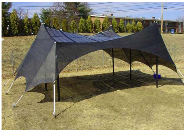
Figure 4. Military tent on which solar energy cells are integrated [11]
