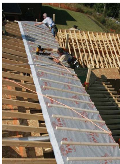
Figure 2: The application of Tyvek brand roofing underlayment [9]
