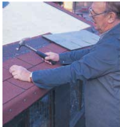
Figure 5: Application of shingle
