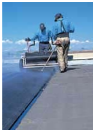
Figure 9: Application of bituminous membrane on a roof
